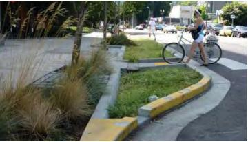
Integrated stormwater filtration planter
