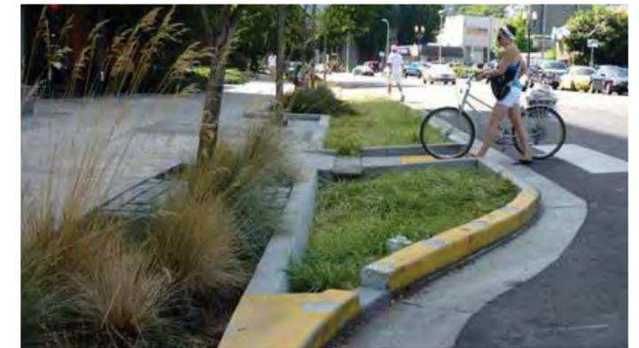
Integrated stormwater filtration planter
